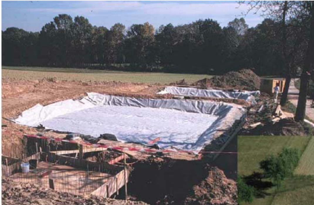
Construction of CW with impermeable synthetic liner
