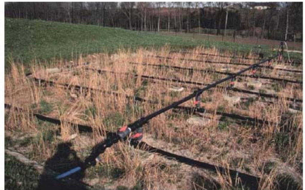
Distribution system of a 40 PE vertical flow plant
