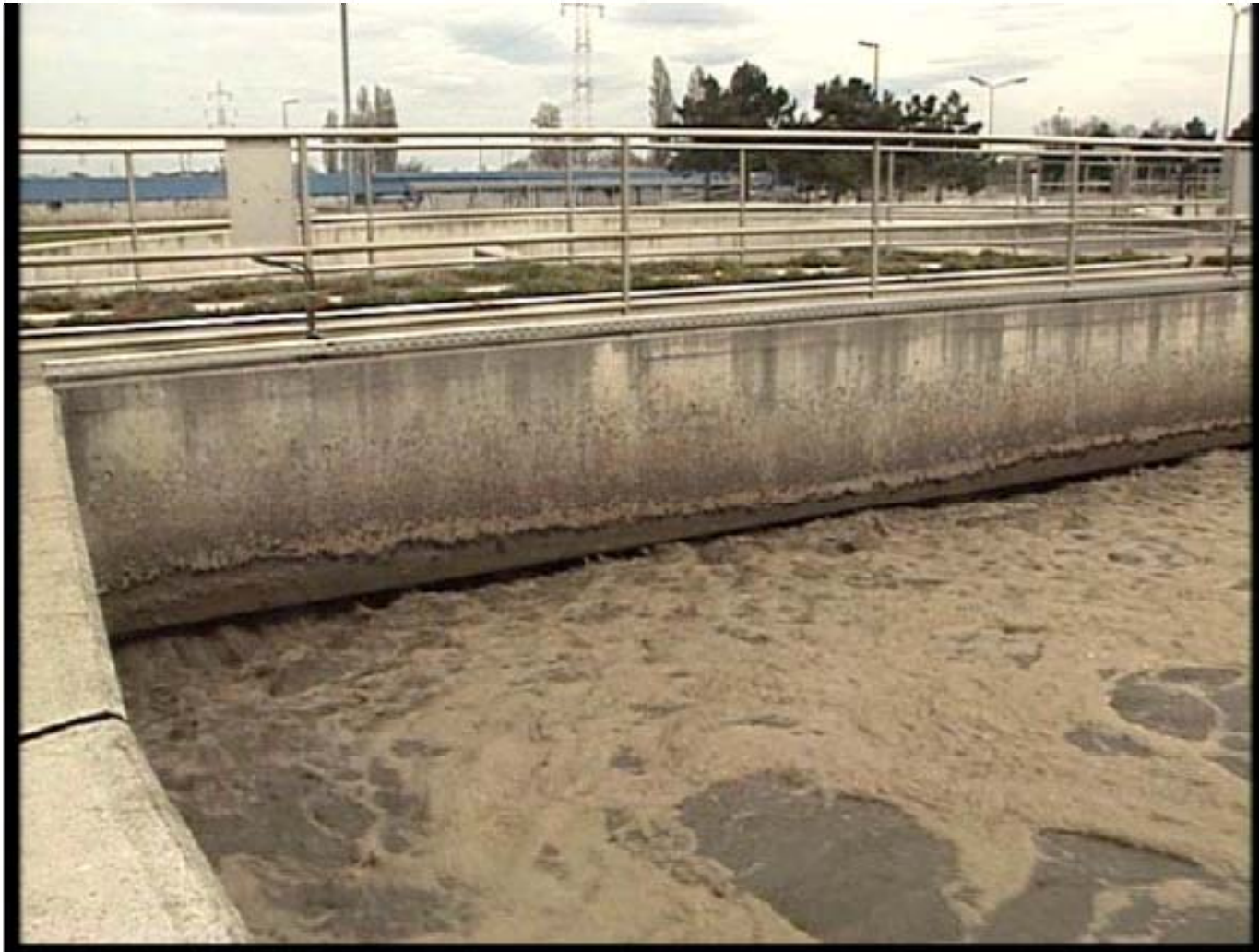
Activated sludge tank with covered cylinder aerator
