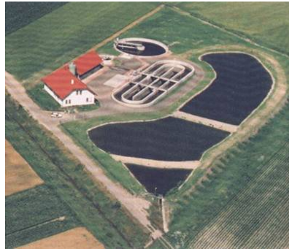
Communal Infrastructure Water / Wastewater
